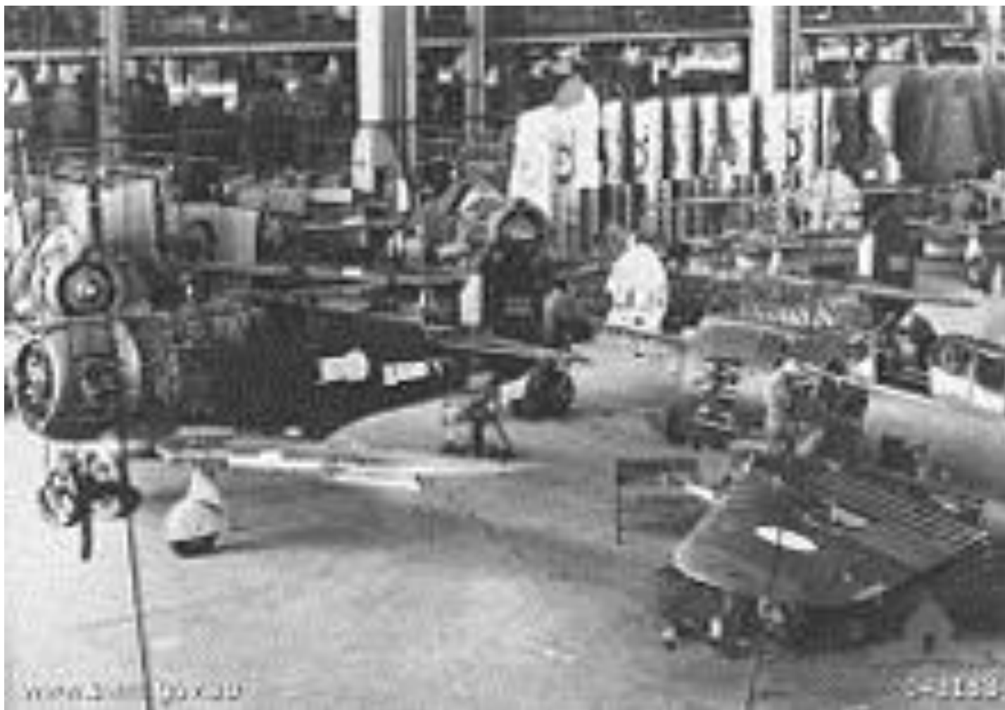
Boomerangs under construction at CAC's factory at Fishermans Bend
